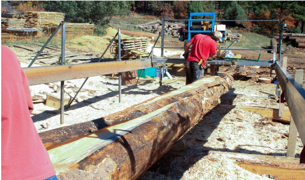
Exhibit 4. Construction Site in the Twin Buttes Development
